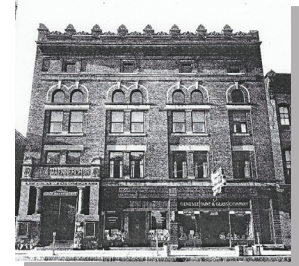
1902 BUILDING- AFTER FIRE, INCORPORATING THE 1893 ENTRY
