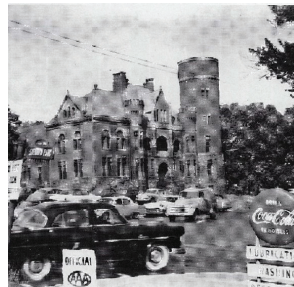
STEUBEN ARMORY PRIOR TO DEMOLITION, 1956
