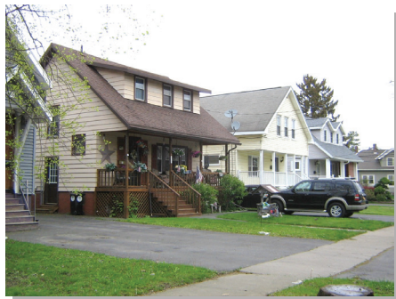
TYPICAL HOMES IN THE NEIGHBORHOOD; THESE ARE ACROSS THE STREET FROM THE CONSTRUCTION
