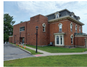
VIEW FROM THE SOUTHWEST
