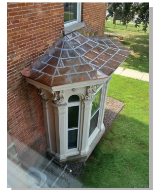
NEW COPPER ROOF ON THE WEST-FACING BAY WINDOW
