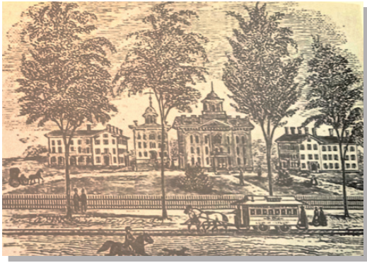
THE WHITESTOWN SEMINARY, MAIN STREET, WHITESBORO (ONEIDA COUNTY HISTORY CENTER/THE HISTORY OF ONEIDA COUNTY, 1977). THE COMPLEX WAS ADAPTED FOR INDUSTRIAL USE IN THE 1890S. TODAY, A PORTION OF THE CENTRAL STRUCTURE REMAINS, ALBEIT HEAVILY MODIFIED.
