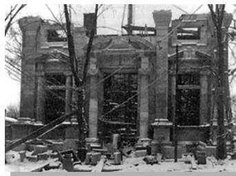
GENESEE STREET FAÇADE UNDER CONSTRUCTION
