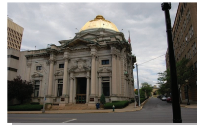
THE 1929 ADDITION AT LEFT WITH 1979 ANNEX AT FAR LEFT
