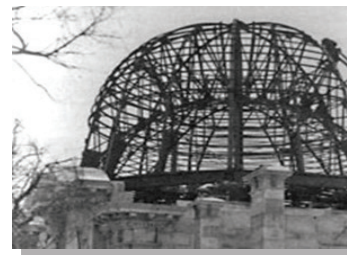
THE DOME UNDER CONSTRUCTION
