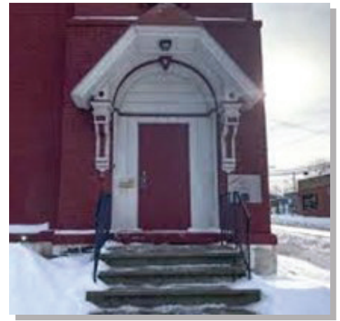
MAIN HALL VARICK ST. ENTRANCE CANOPY WITH CONSOLES
