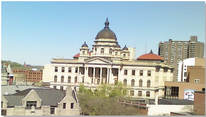
A VIEW FROM THE EDITOR'S OFFICE WINDOW IN THE GALLERIES OF SYRACUSE OF THE ONONDAGA COUNTY COURT HOUSE ON COLUMBUS CIRCLE, DESIGNED BY ARCHIMEDES RUSSELL (1904-07).
